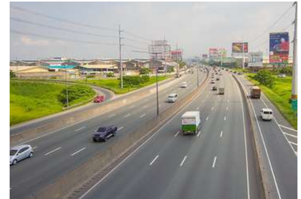
North Luzon Expressway
